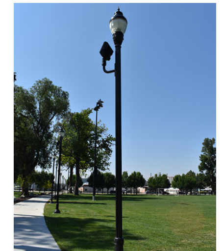
S3. Single light pole - ornate with solar panel
