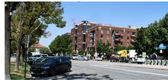
X1. North end, 300 South (looking northwest)
